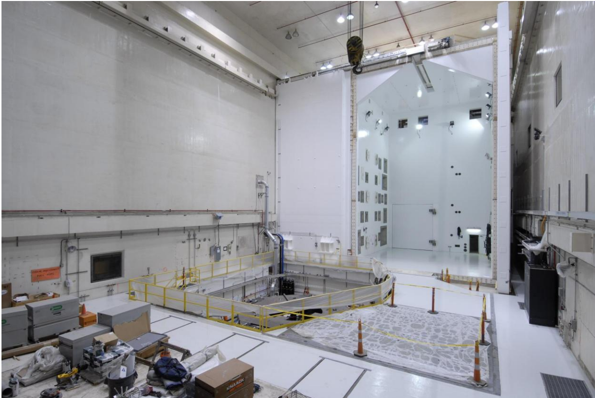
Figure 11: Construction photo taken 26 November 2010 showing the interior view of the RATF chamber; also visible is the SET mechanical vibration facility (mid-left, below surface level) and the modal test floor (mid-right)
