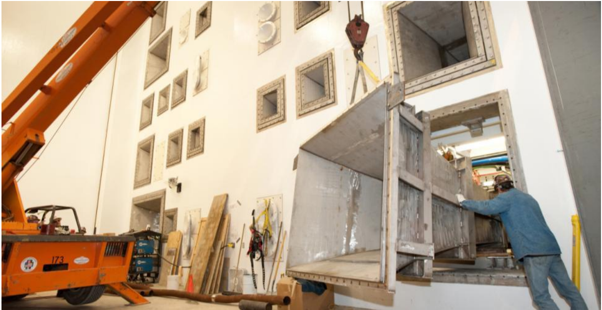
Figure 7: Construction photo showing the installation of the final RATF horn (25 Hz)
